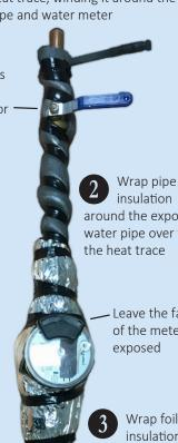
around the exposed water pipe over top the heat trace
