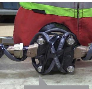
**PRO TIP! Apply the heat** trace in a criss-cross pattern under the water meter
